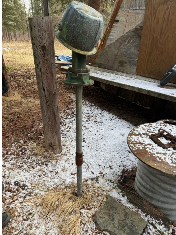
Figure 12. Groundwater Well at Home #2
