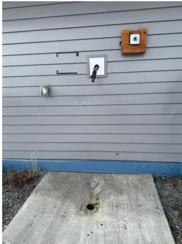
Figure 2. Water hauling point at the Utility Building
