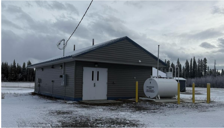
Figure 1. Water facility Building
