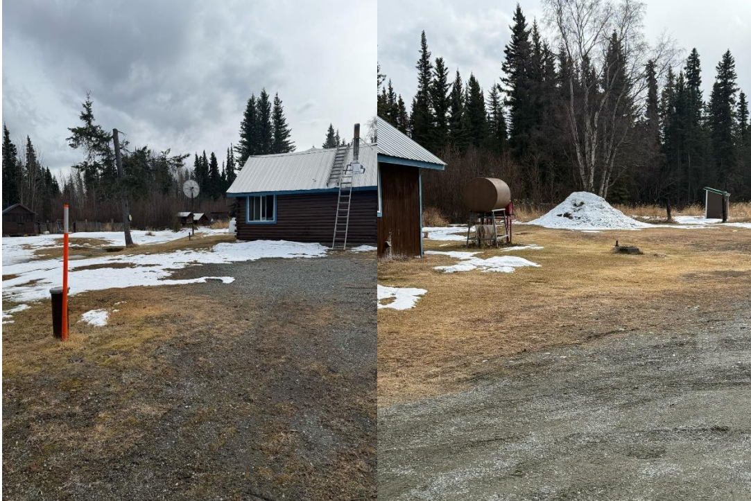
Figure 17. Home #12 groundwater well and septic system
