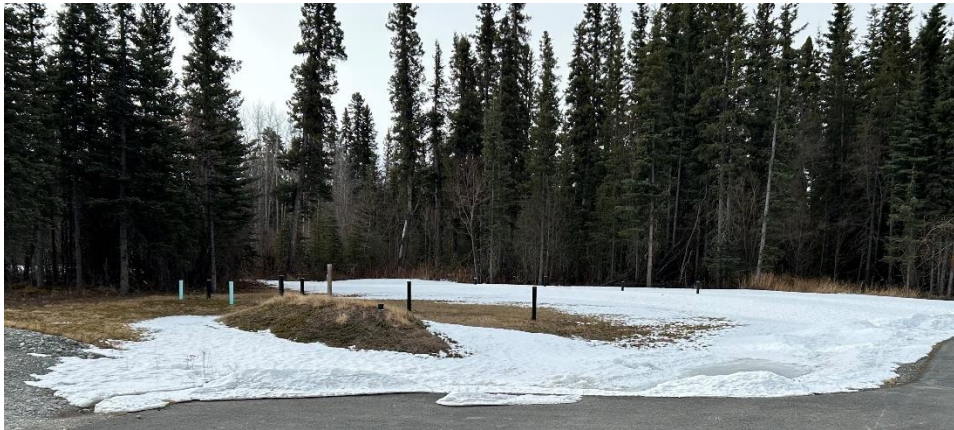
Figure 11. Septic system for clinic (not evaluated as part of this PER)
