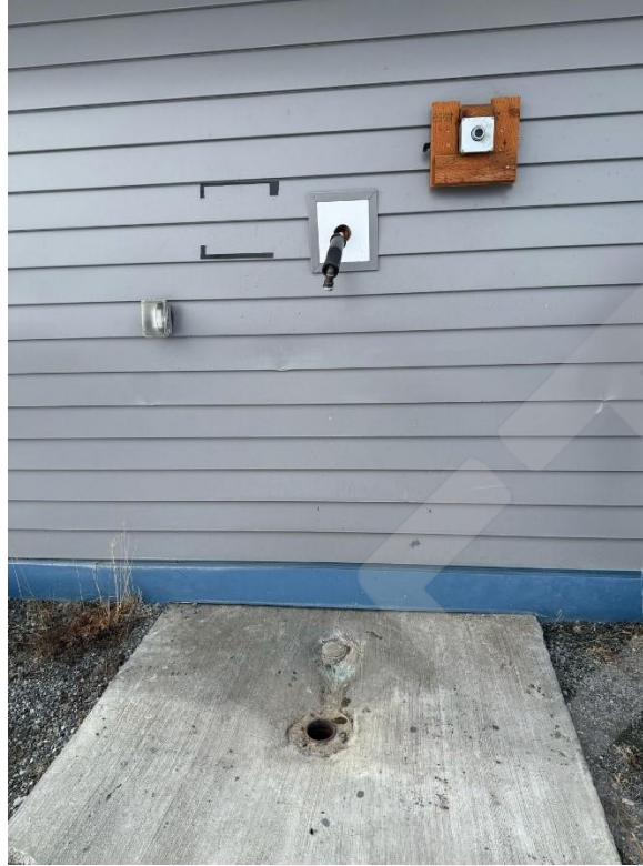
Figure 7. Water hauling point at the Utility Building
